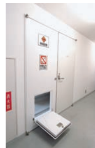
設置後 After installation
